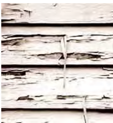
Extensively deteriorated paint needs to be removed to bare wood, then primed and repainted. Photo: NPS files.
