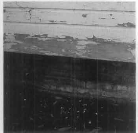
Figure 7. Chalking exterior paint can cause dangerous lead levels in soil around a house. Lead levels are usually highest in the one foot wide area adjacent to the building foundation. In these cases, the existing soil should be replaced with new soil or sod. This is particularly important if children and small pets play in contaminated areas, then inadvertently track the dirt inside.
