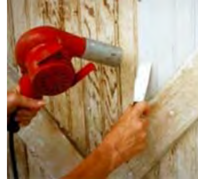
The nozzle on the electric heat gun permits hot air to be aimed into cavities on solid decorative surfaces, such as this carriage house door. After the paint has been sufficiently softened, it can be carefully removed with a scraper. Photo: NPS files.
