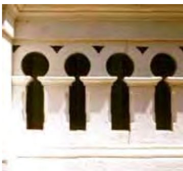
The paint on this exterior decorative feature is sound. Photo: NPS files.
