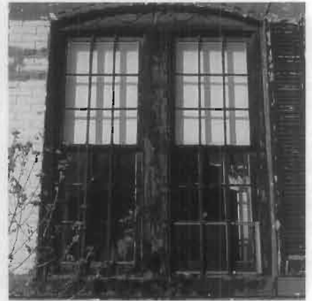
Figure 6. Deteriorating operable windows often contribute to lead dust in a house. Peeling paint and small particles from abraded surfaces collect in window troughs or sills and are then carried inside by air currents, settling on floors. When the lead dust mixes with regular house dust, it can easily be ingested by a child through hand to mouth contact. In homes with small children, floors and other surfaces should be kept as clean as possible to avoid lead contamination.
