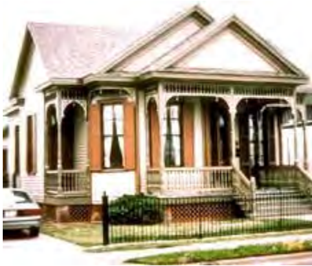
Decorative features were painted with a traditional oil-based paint as a part of the rehabilitation. Photo: NPS files.
