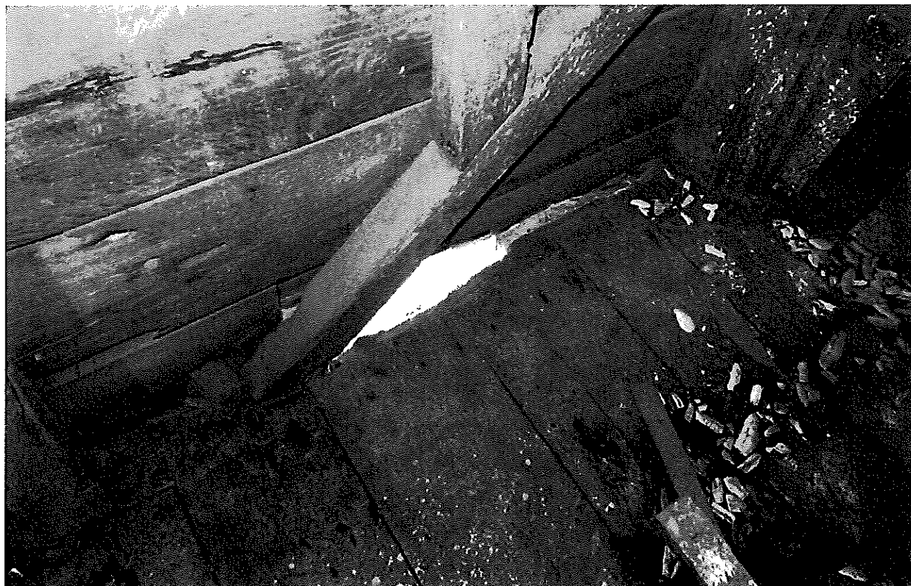
S-1 Deteriorated sill, north-east corner (2017)
