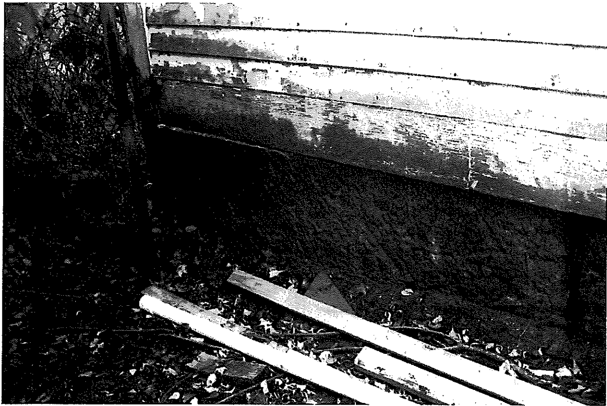
S-1 Shifting at foundation below sill, north-west corner (2013)
