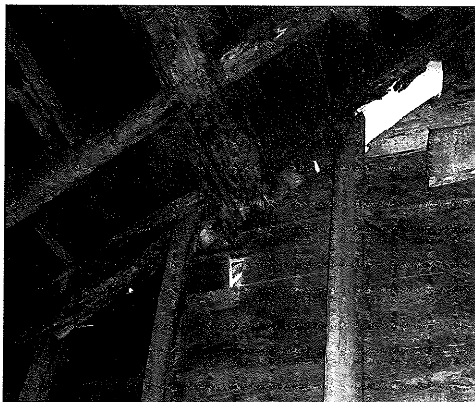
S-3 Deteriorated rafter and purlin connection on east slope of north wall with shoring (2017)
