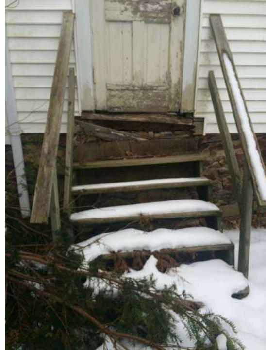
Figure 7: West Stair - Failed Connection
