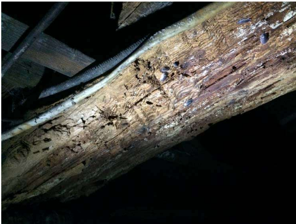
Figure 15: Basement - ±15' Northeast of Southwest Building Corner - Severely Deteriorated Beam
