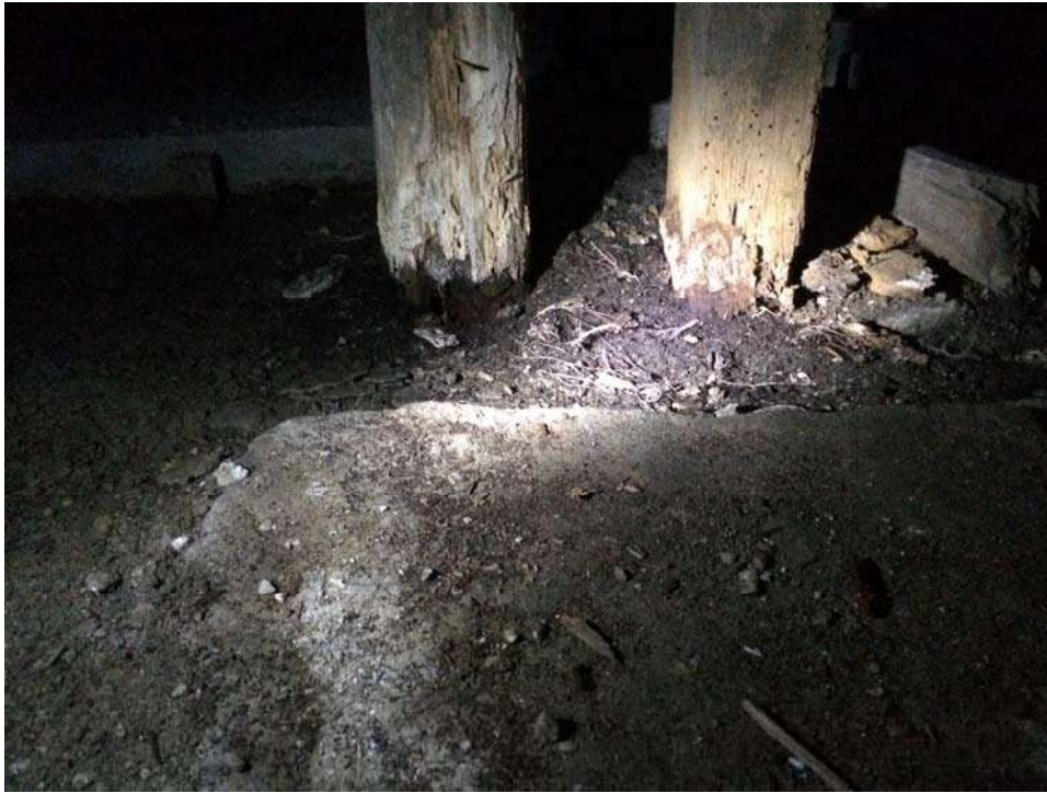
Figure 14: Basement - Decayed Column Bases, Typical Condition
