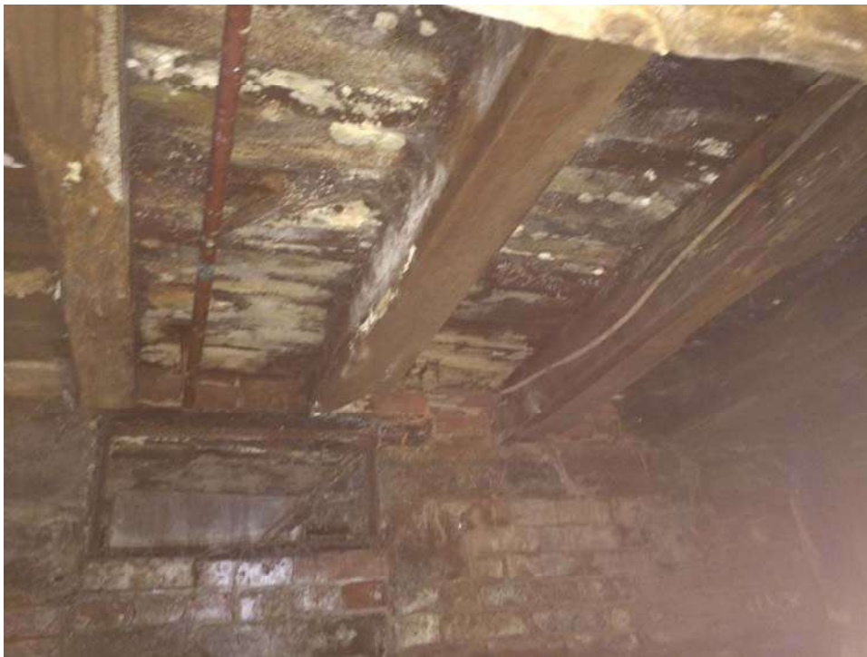
Figure 18: Basement – Looking South Toward South Wall - Mold Growth
