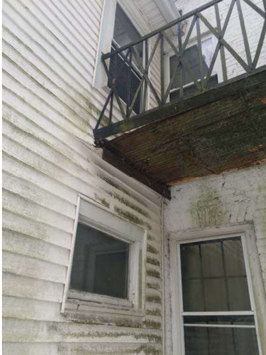
Figure 6: West Face Escape - Failed Connection
