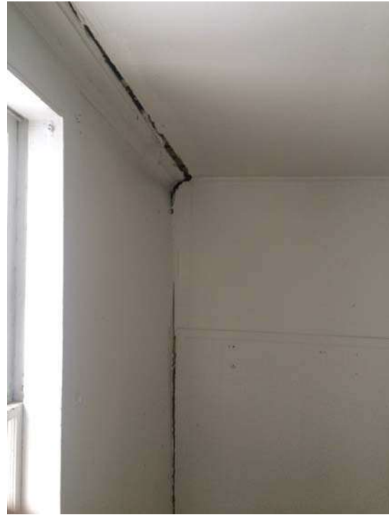
Figure 9: Roof to Wall - Unit 5 - Rafter Lateral Failure
