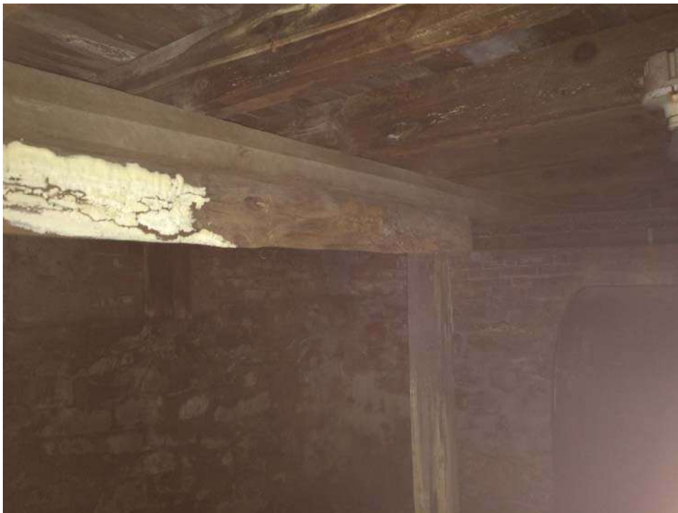
Figure 16: Basement – Looking Southwest Toward Southwest Corner - Mold Growth
