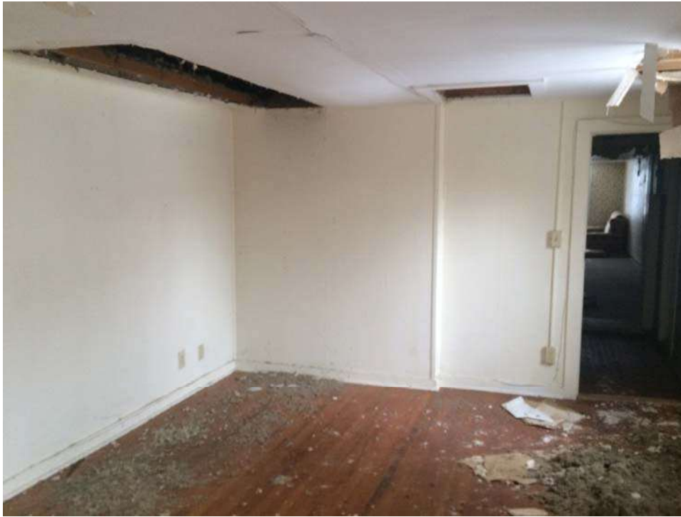
Figure 19: Unit 5 Looking South, Water Damaged Ceiling
