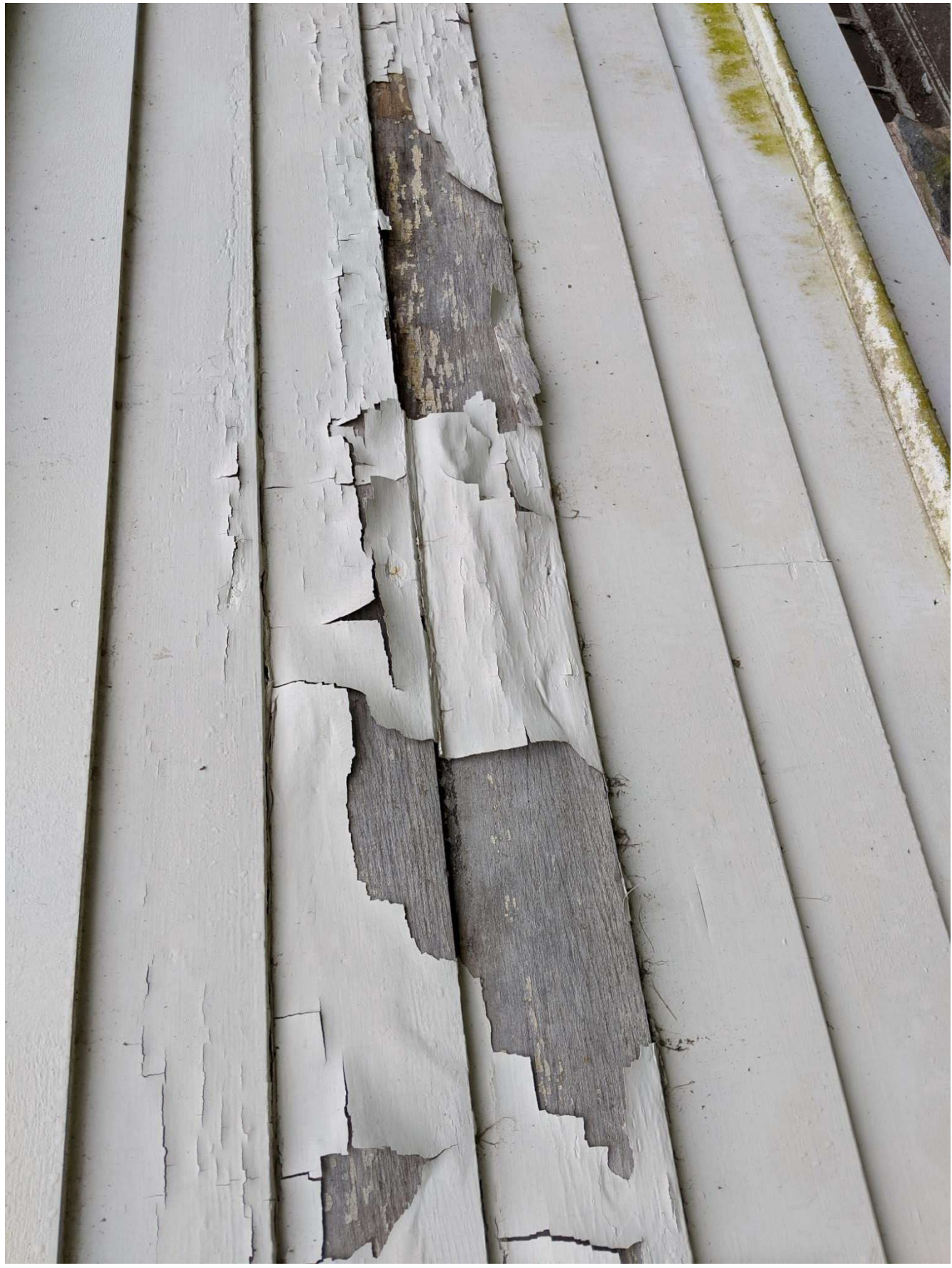
Photograph 6: Eli Whitney Boarding House (1827) detail of northern elevation peeling.
