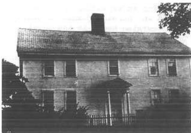
10: Early Georgian house on Harvey Road, Stonington.
